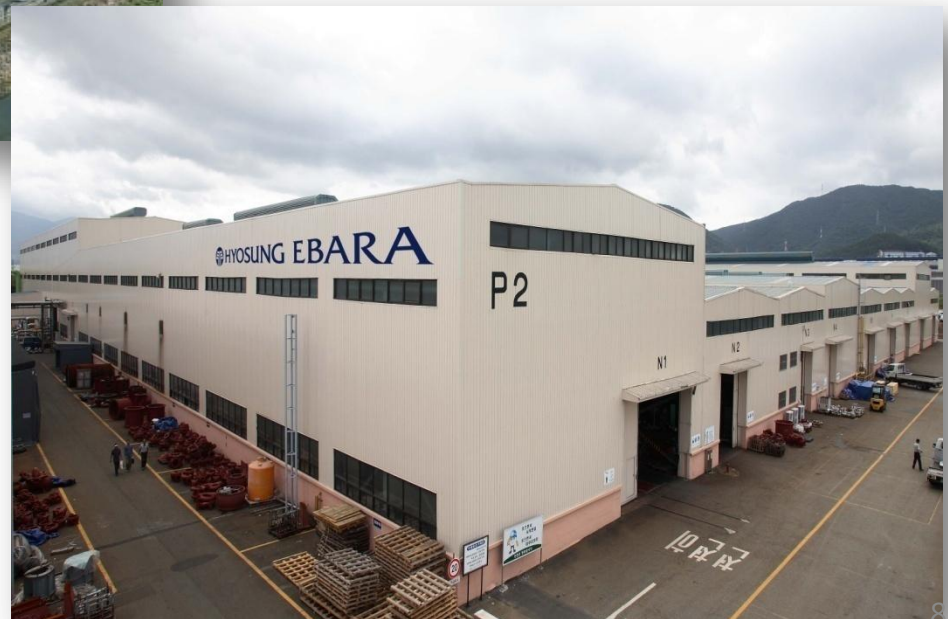
Hyosung Ebara PU (Assembly Line)
