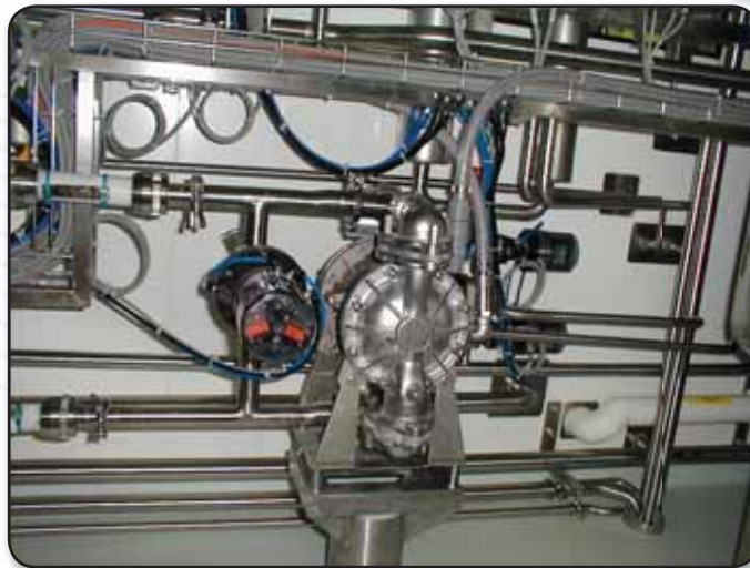
USDA certified ball check valve pump in a clean-in-place, sanitary piping installation.
