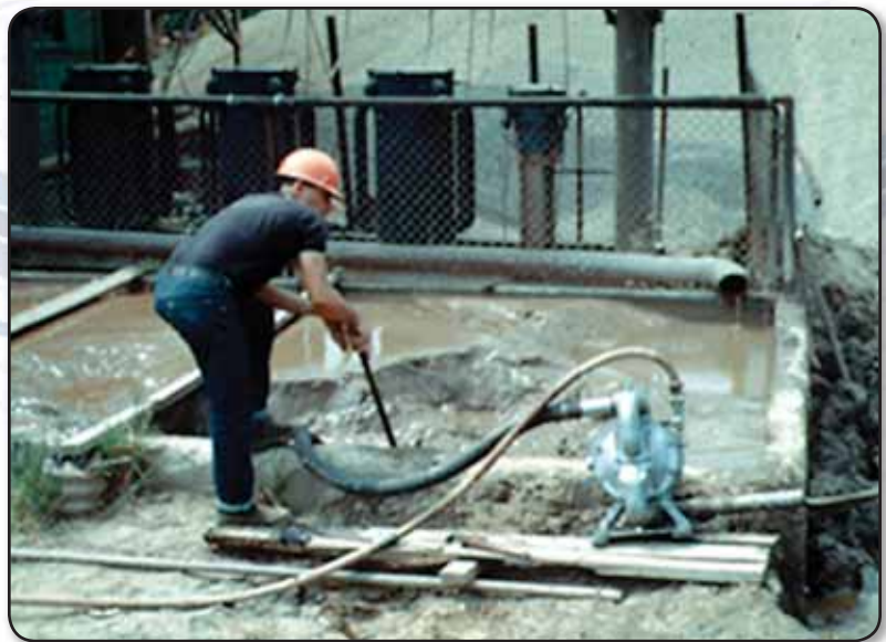
Heavy duty flap valve pump temporarily installed pumping settling pond sludge. (Perfect alignment not required).
